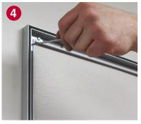
Tip: Adjust corner clips if needed to achieve plumb corners before putting in screws.
